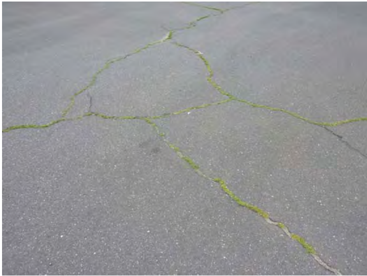
Typical cracking of asphalt paving in project drive.
