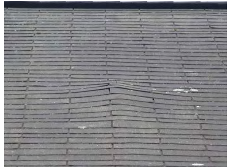
Localized roof sheathing substrate failure. Asphalt roofing shingles are shown to be replaced early in the term.
