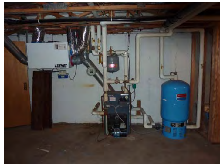
Abandoned white heat recovery system, Boiler, and blue domestic hot water tank in basement is typical for each apartment.
