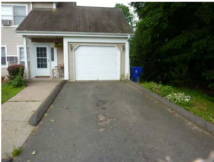
Asphalt failure in unit driveway. Asphalt curb is one of several typical trip hazards shown to be eliminated in Year 1.
