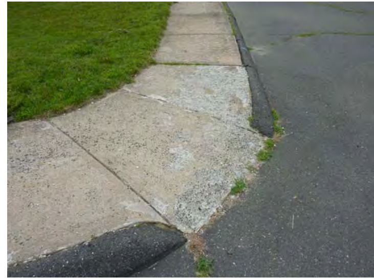
Asphalt curb and concrete walk damage from snow removal is shown to be repaired in Year 1.
