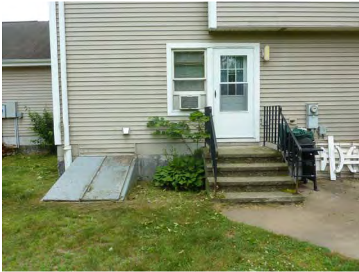
Riser height varies at concrete stair and is a typical trip hazard shown to be eliminated in Year 1. Concrete stoop, handrail and basement hatch and windows are all shown to be replaced in Year 1.
